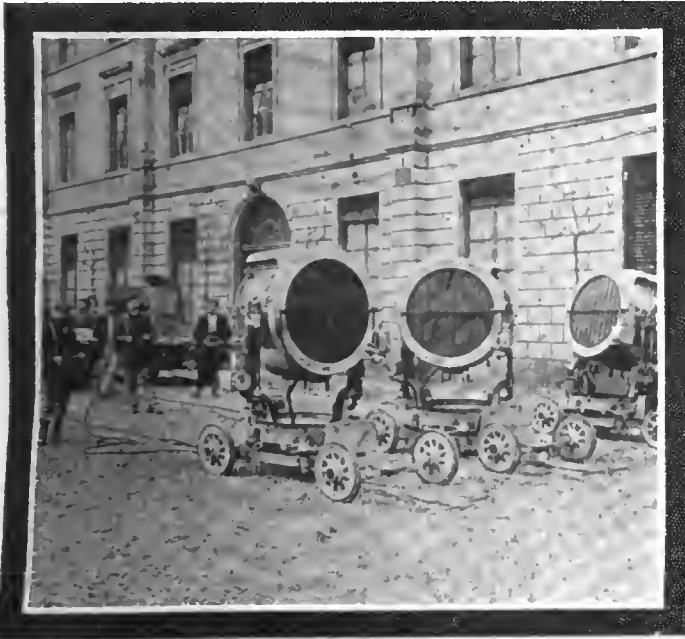
Projectors in position for operation. Compressed air control
